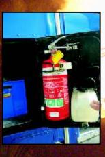
The pin has to be unobstructed with no visible damage. The alignment of the pin and its bracket holder has to be precise.
